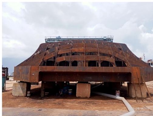
Gambar 2.32 Inspect fit up frame
