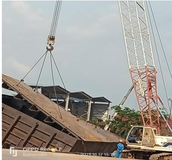
Gambar 2.74 Erection main deck
