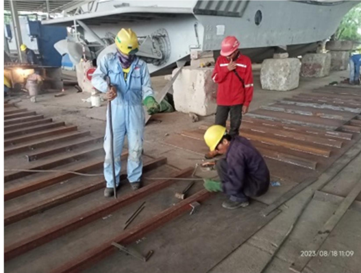
Gambar 2.33 Fit up deck house
