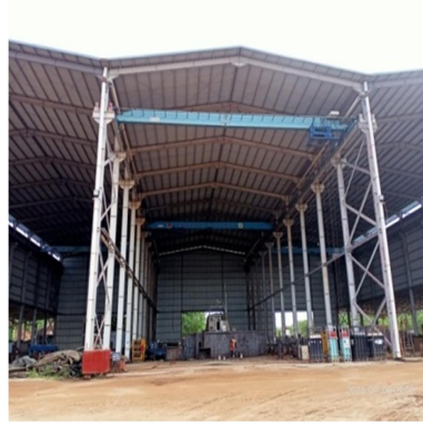
Gambar 1.4 Main Workshop Fabrication
