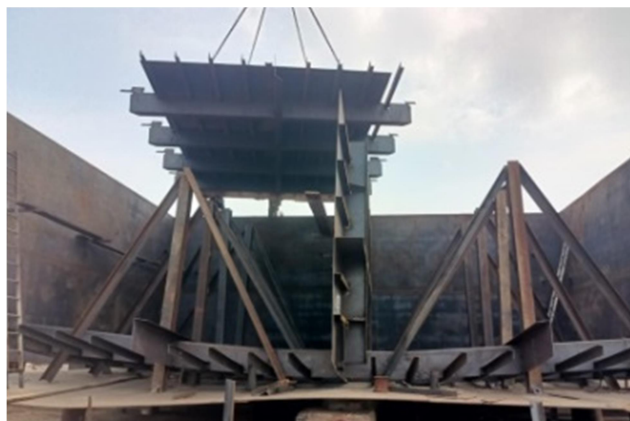
Gambar 2.73 Fit up main deck
