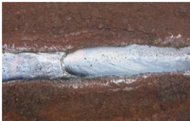
Gambar 3.21 Penampalan kebocoran
