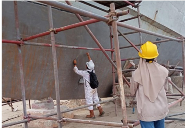
Gambar 2.47 inspection after blasting
