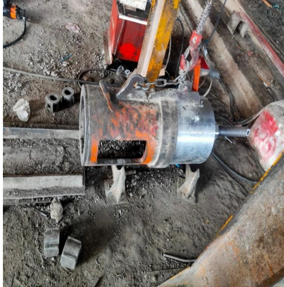
Gambar 3.37: Mesin Stressing
