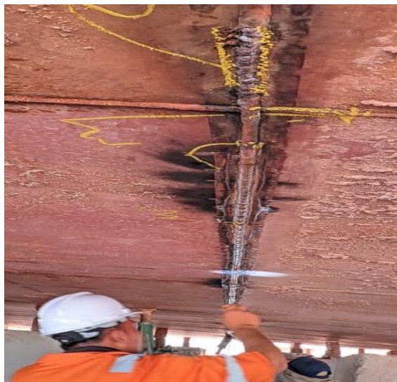
Gambar 2.85 Gambar proses pengecekan beking cramik
