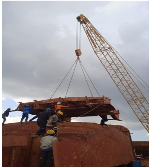
Gambar 2.147 Erection Engine Girder
