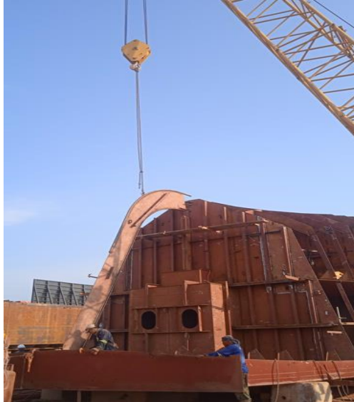
Gambar 2.139 Erection Girder keel
