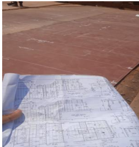
Gambar 2.138 Pengecekan markingan Bridge House
