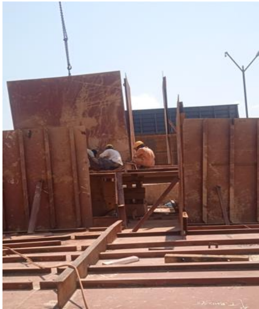
Gambar 2.141 Erection Bridge Deck
