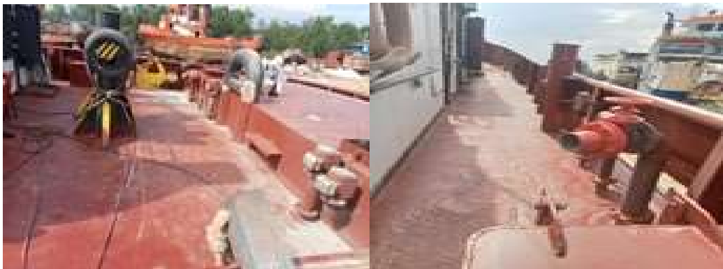
Gambar 3.26 Pengecatan Anti Corrosive ( Area Main Deck-Internal Bulwark )
