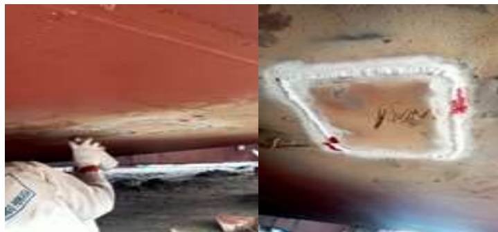
Gambar 2.102 Proses Penetran Test Kamar Mesin OWS
