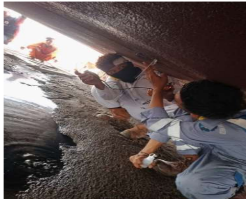
Gambar 2.23 Proses Ultrasonic Thickness Test Gauge
