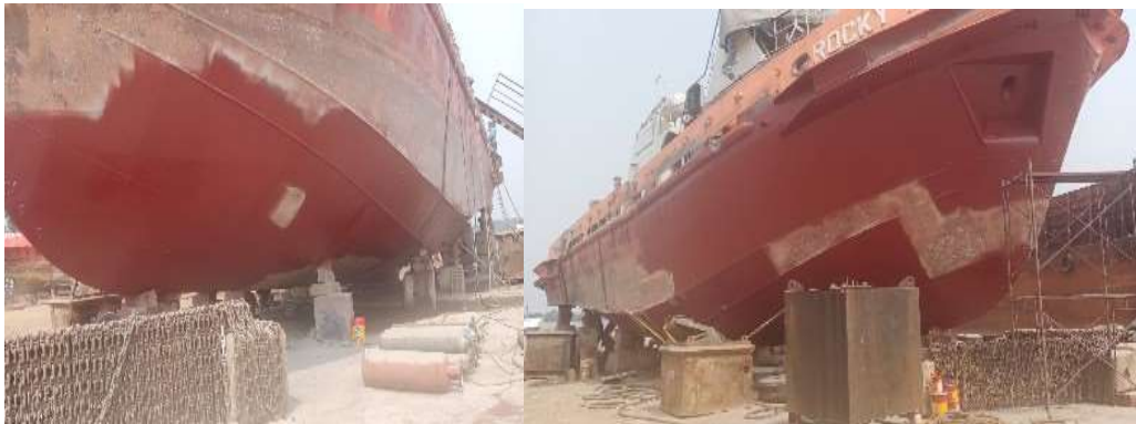
Gambar 3.25 Pengecatan Anti Corrosive ( Area Underwater-Topside )
