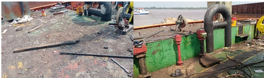
Gambar 3.15 Area Main Deck
