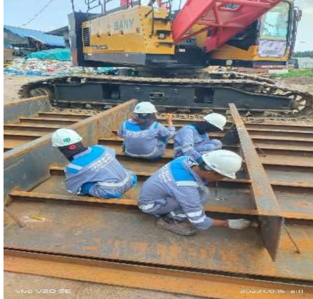
Gambar 2.16 Checking Weld Defects
