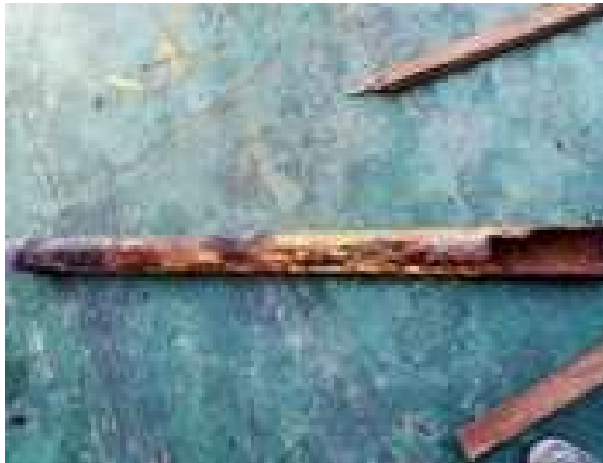
Gambar 2.118 Pemotongan Pipa Scupper
