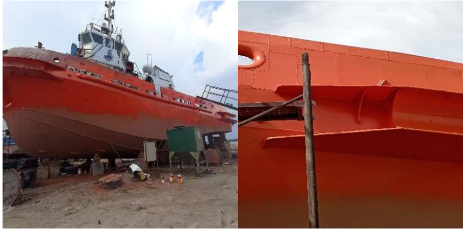
Gambar 2.85 Pengecatan Second Coat Topside-Bulwark
