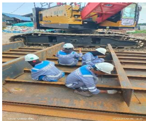
Gambar 2.22 Checking Weld Defects
