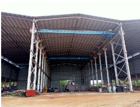
Gambar 1.3 Main Workshop Fabrication
