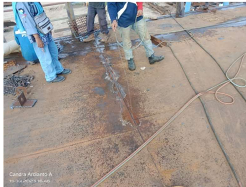
Gambar 2.11 Control proses air test Tengki Tongkang ( H.169 Sorento Bay )
