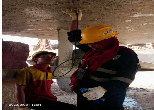
Gambar 3.2 Proses pengujian Ultrasonic Thickness Test
