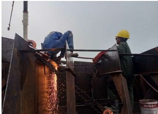
Gambar 2.67 Fitting web buritan T.037 Grando Dolphin
