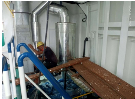
Gambar 2.14 Control fitting ducting coferdam T.027 Marino Dolphin
