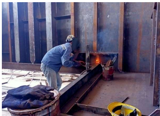
Gambar 2.33 Control Weldingan Bracket Deck House T.036 Louis Dolphi
