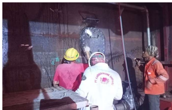
Gambar 2.89 Air test tanki T.033 JX walrus
