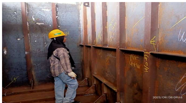
Gambar 2.54 Inspek Visual Test Deck House T.033 Jx Walrus
