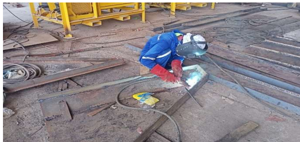
Gambar 2.77 Control welding Mast Foundation T.033 Jx Walrus
