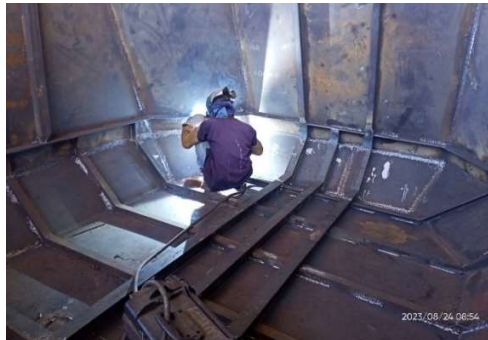
Gambar 2.41 Control Welding Well House T.036 Louis Dolphin
