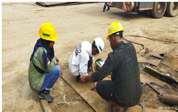
Gambar 2.87 Marking Bracket web T.037 Grando Dolphin
