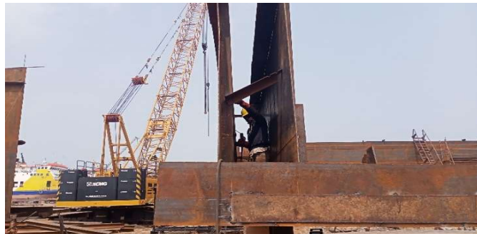
Gambar 2.65 Control welding BHD Haluan T.037 Grando Dolphin
