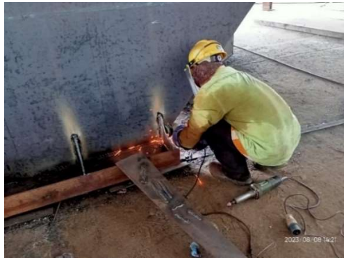
Gambar 2.31 Control Grinding Bracket Deck House T.036 Louis Dolphin
