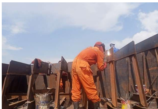
Gambar 2.68 Control Welding web buritan T.037 Grando Dolphin
