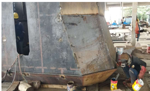
Gambar 2.70 Control Welding deck house t.037 Grando Dolphin
