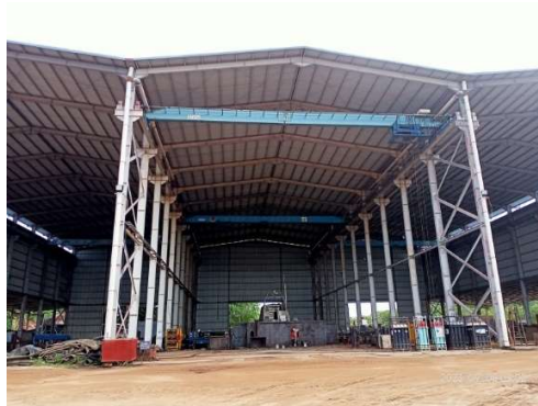
Gambar 1.3 Main Workshop Fabrication
