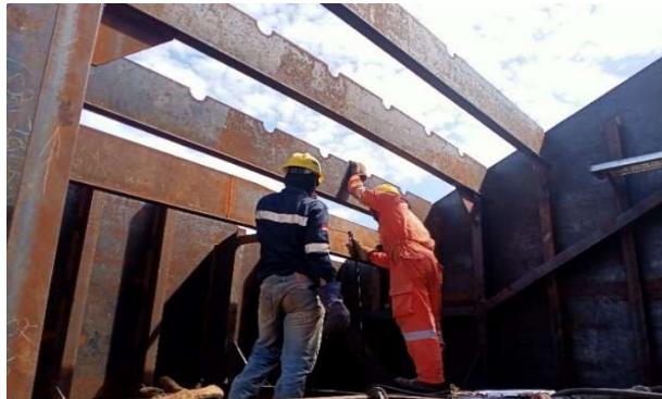
Gambar 2.43 Control instal Web Frame T.033 Jx Walrus
