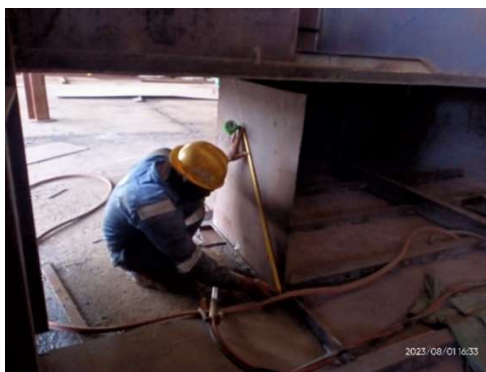
Gambar 2.25 Fitting Deck House frame 23 -25 T.036 louis Dolphin
