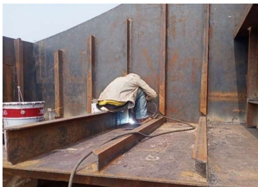
Gambar 2.64 Control welding long BHD T.037 Grando Dholphin
