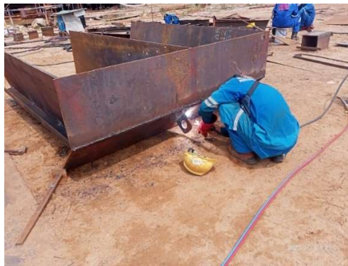
Gambar 2.75 Welding Chain Locker T.036 Louis Dolphin
