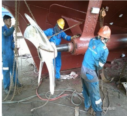
Gambar 3.1 28.finishing propeler
