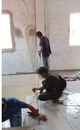
Gambar III.124 Marking As (Sumber: Dokumentasi Lapangan 2023)
