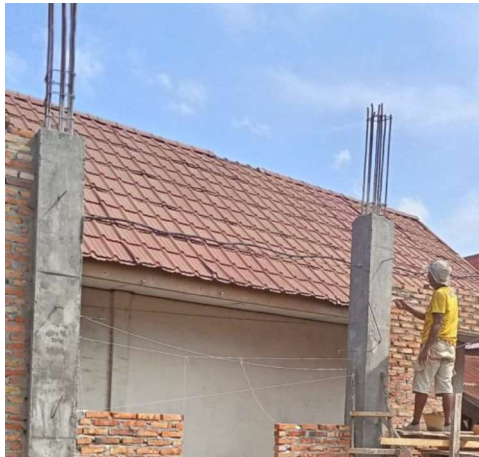
Gambar III.30 Marking Titik As (Sumber: Dokumentasi Lapangan 2023)
