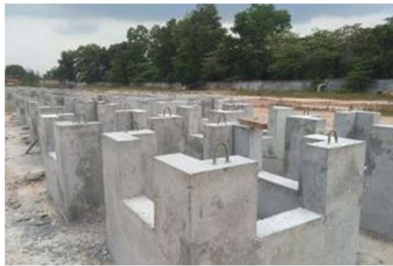
Gambar 2.4 precast pile cap
