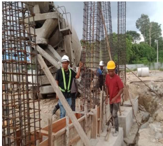
Gambar 3.25 pengecoran tie beam
