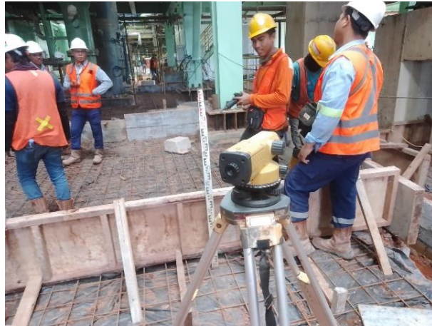
Gambar 2.10 Marking Topcor Lantai Man Power House (MPH) Grid 4-5 Sumber : Dokumentasi lapangan, 2023
