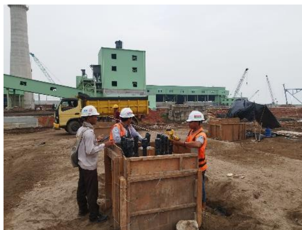
Gambar 3.12 Marking as anchor Sumber : Dokumentasi Proyek, 2023
