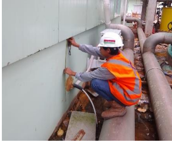
Gambar 2.14 Marking Aprone Cemical Water Tritmen (CWT) Sumber : Dokumentasi lapangan, 2023
