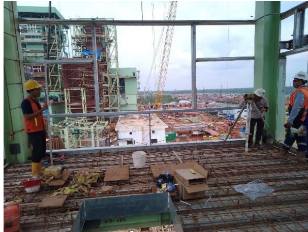
Gambar 2.12 Join inspection top cor M2transfer tower Sumber : Dokumentasi lapangan, 2023
