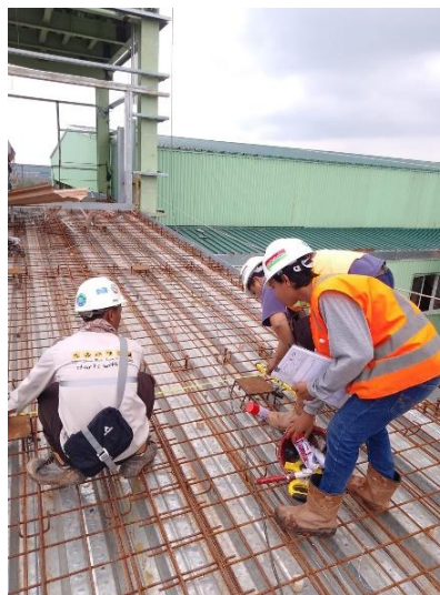
Gambar 2.15 Join Inspection Embeded M2 Trstle Sumber : Dokumentasi lapangan, 2023
