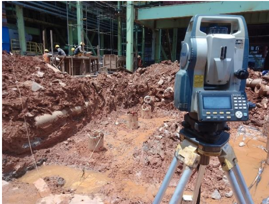
Gambar 2.16 Marking Top Lean Cocrate(LC) Id Fan Of Boiler #2 Sumber : Dokumentasi lapangan, 2023
