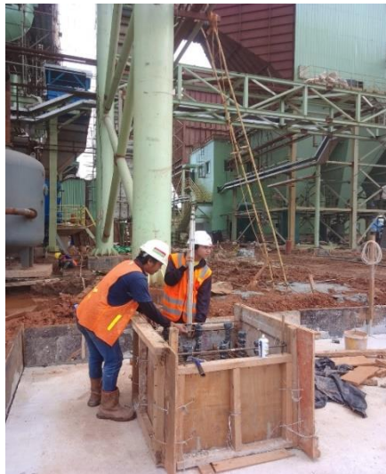
Gambar 2.9 Marking Top Cor (TOC) Pedestal Slag Transmission Station Sumber : Dokumentasi lapangan, 2023
