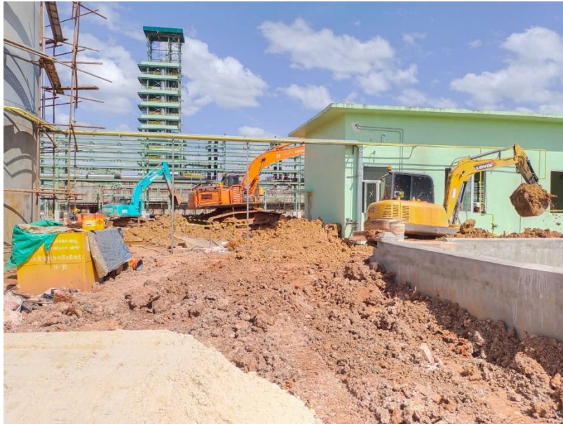
Gambar 3.13 Penimbunan Tanah Area Oil pump House (Sumber: Dokumentasi lapangan 2023)
