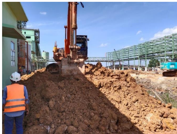
Gambar 3.12 Penimbunan Tanah Area Oil pump House
