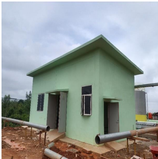
Gambar 2.27 . Oil Pump House
