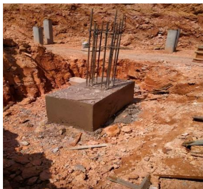
Gambar 3. 4 Kolom Pedestal
