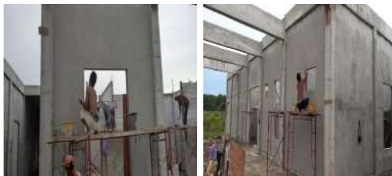
Gambar 3.14 21 Pekerjaan acian dinding.
