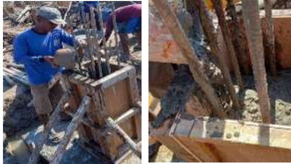
Gambar 3.14 3 Pengecoran Kolam Pedestal
