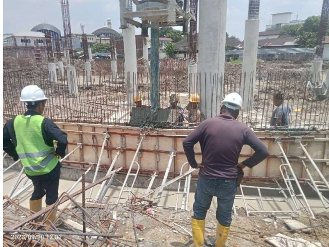
Gambar 3.52 Pengisian bekisting dan vibrator beton concrete f'c 25
