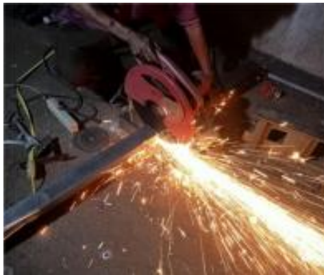
Gambar 4.9 Cutting (Pemotongan Besi UNP)
