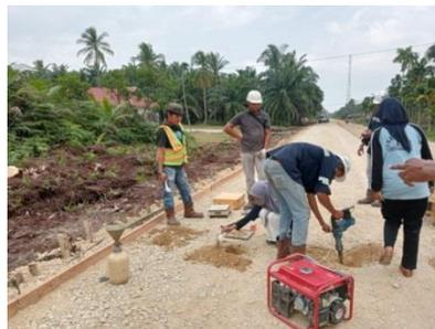
Gambar 3. 21 *Coredrill Base*
