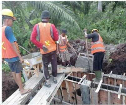
Gambar 3. 5 Pengecoran Dinding Turap
