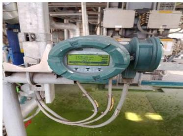
Gambar 2. 6 Temperatur Transmitter
