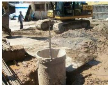
Gambar 3.15 Casing temporary
