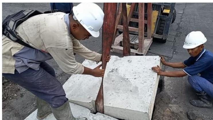
*Gambar 3.10 Erection Penutup Drainase
