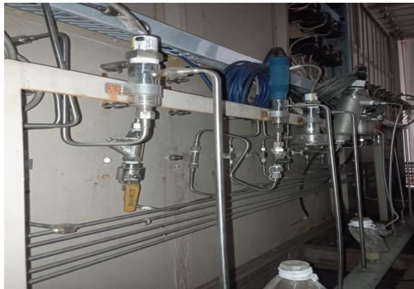
Gambar 2. 2 Pergantian pipa turbin
