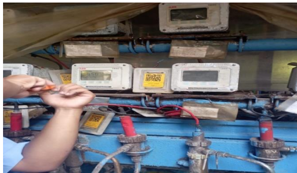
Gambar 2. 5 Pembongkaran transmitter conduct
