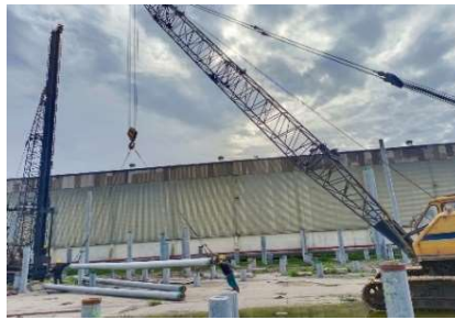
Gambar 3.9 Kegiatan Mobilisasi Lifting Spun Pile
