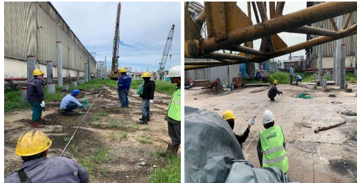
Gambar 3.5 Kegiatan Pengukuran Stake Out
