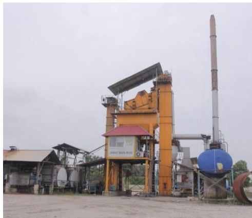
Gambar 3. 12 Asphalt mixing plant Sumber : Dokumentasi lapangan,2023
