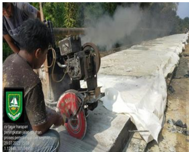
Gambar 3.16 Cutting Beton
