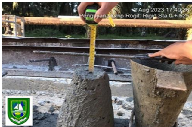
Gambar 3.12 Pengujian Slump Test Rigid.
