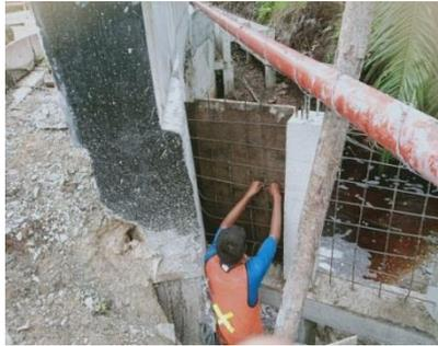
Gambar 3. 3 Pemasangan Bekisting Turap
