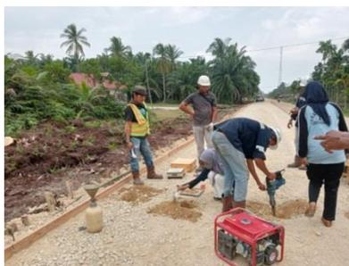
*Gambar 3. 19 Coredrill Base
