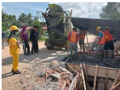
*Gambar 3. 14 Pengecoran Box Culvert*
