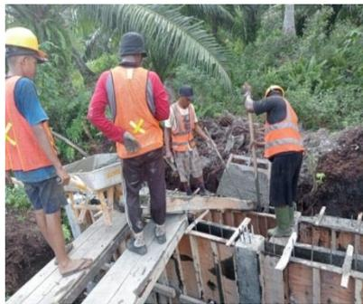
Gambar 3. 4 Pengecoran Dinding Turap
