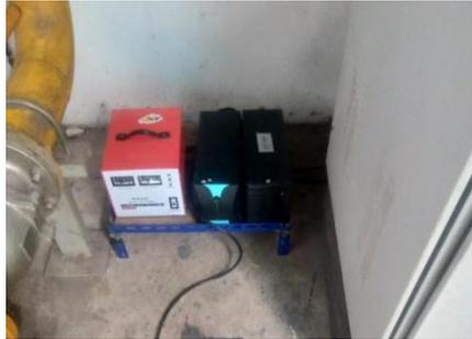
Gambar 2.6 UPS (Uninterruptible Power Supply)
