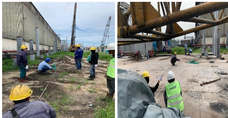
Gambar 3.5 Kegiatan Pengukuran Stake Out
