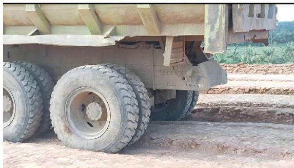
Gambar 3. 32 uji proof rolling tanah
