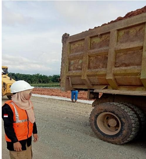
Gambar 3. 34 uji proof rolling Lapisan drainase
