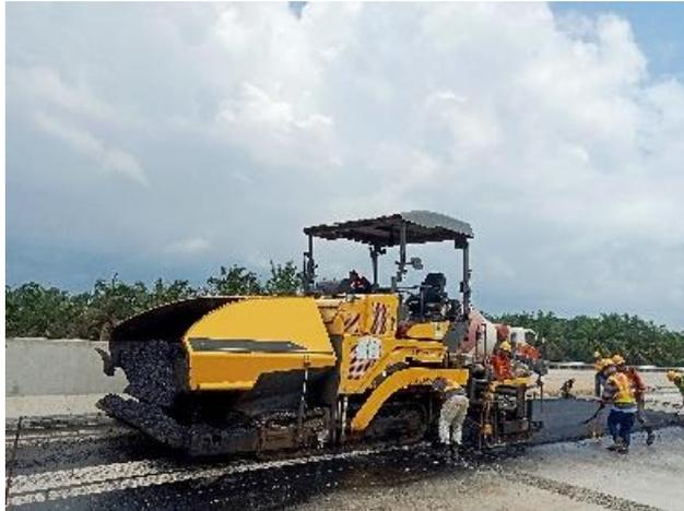
Gambar 3. 14 Asphalt paver
