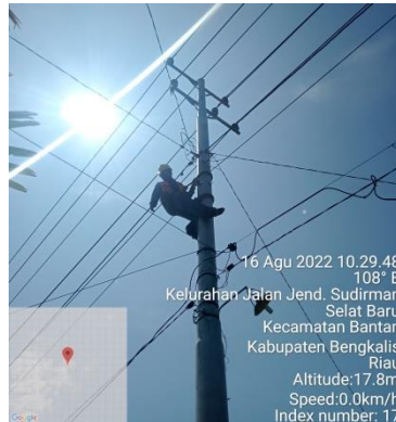
Gambar 2.47. Lost contact (Sumber: PT. Adra Gemilang)
