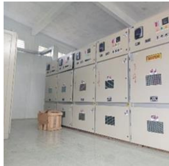
Gambar 2.19. Monitoring beban feeder (Sumber: PT. Adra Gemilang)
