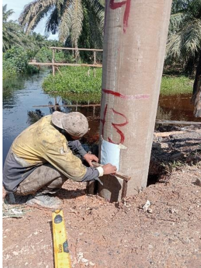
Gambar 4. 9 Calendering Test
