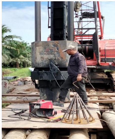
Gambar 4. 4 Pengecekan Hammer Diesel
