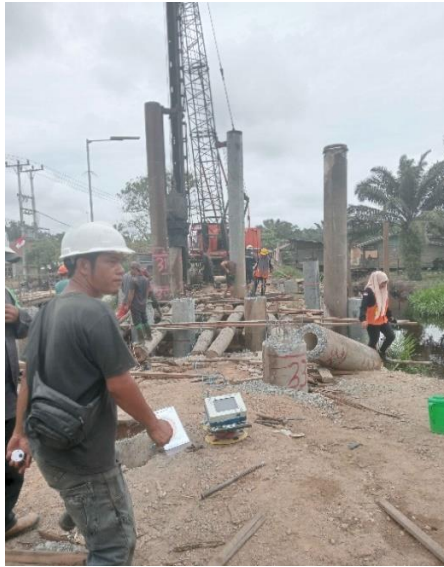
Gambar 4. 10 PDA Test
