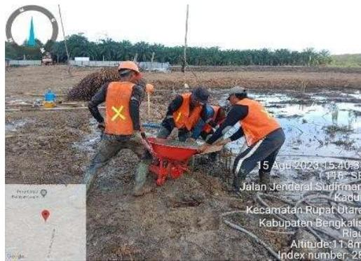
Gambar 3. 11 Proses pengecoran strauss pile
