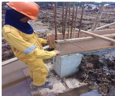
Gambar 3. 30 Mengukur bekisting sloof
