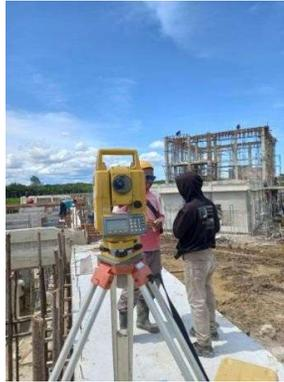
Gambar 3. 50 Pekerjaan survey titik as
