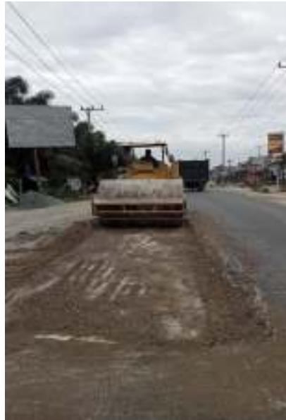
Gambar 3.4 vibrator roller
