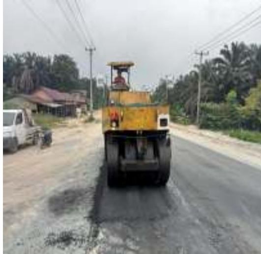
Gambar 3.10 pneumatic tier roller
