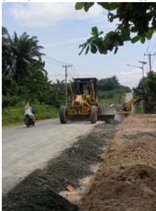
Gambar 3.17 Pehamparan base aggregate kelas A
