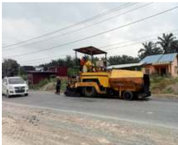
Gambar 3.9 asphalt finisher
