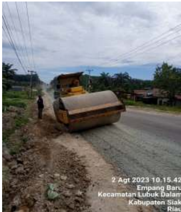
Gambar 4.5 vibrator roller
