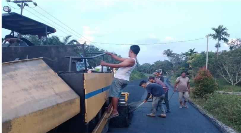
Gambar 3.7. Asphalt finisher
