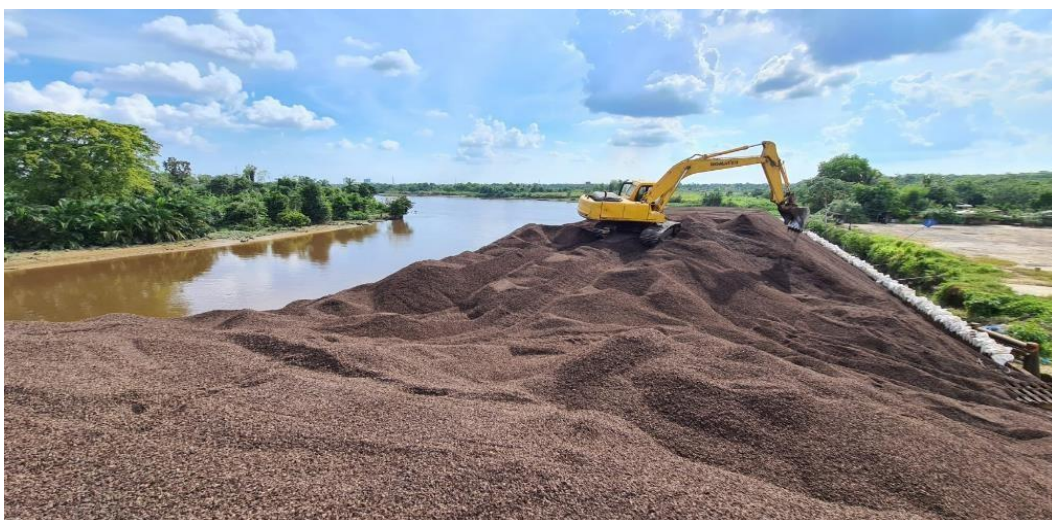
Figure 2.2 Rumbai Stockpile Source: Rumbai Stockpile
