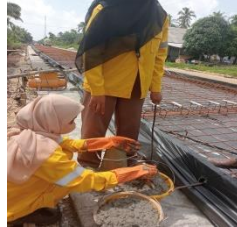
Proses pengujian slump
