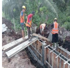
Proses meletakkan campuran beton kedalam bekisting dinding turap
