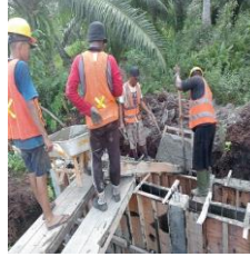
Proses meletakkan campuran beton kedalam bekisting dinding turap
