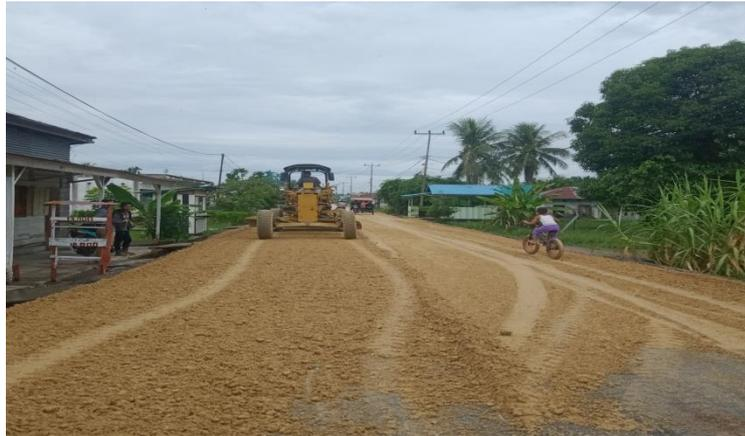
Gambar 3.4 Motor Grader
