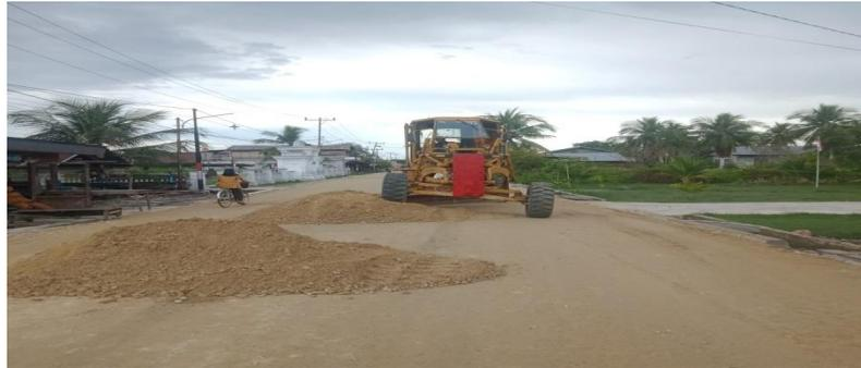
Gambar 4.3 Motor Grader
