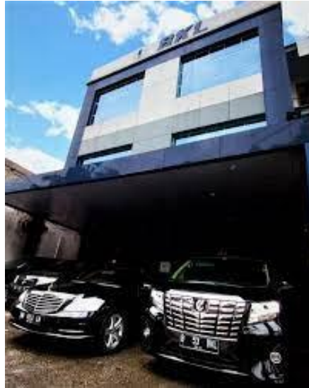
Figure 2.1 The Head Office of BKL Source: Documentation, 2024
