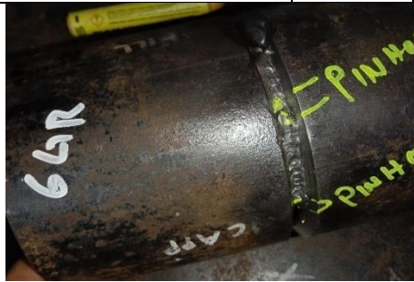
Gambar 4.562 Hasil repair inspeksi visual 6GR Butt joint Sumber: Penulis
