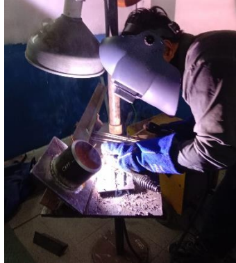
Gambar 4.50 Proses pengelasan dan capping Tee joint
