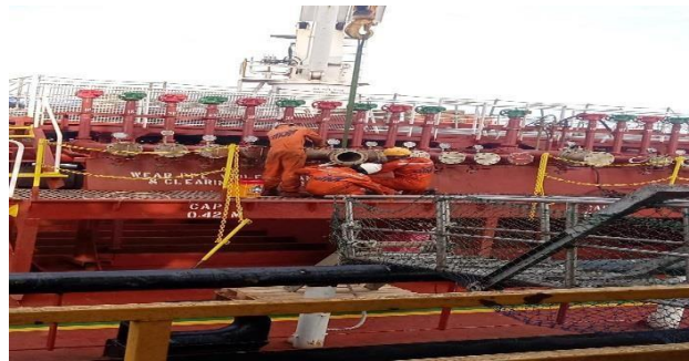
Gambar 3.2 Proses pemasangan reducer
