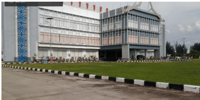
Figure 3.8 Main Office RU II Sources: Processes Data 2024
