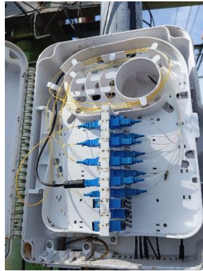
Gambar 3.2 2 Optical Distribution Point
