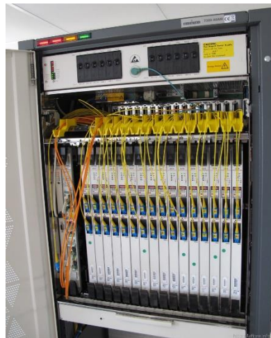
Gambar 3.2 1 Optical Line Terminal
