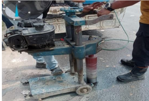
gambar 4. 9 Pengujian Core Drill
