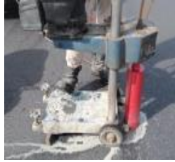
gambar 3. 29 Pengujian core drill lapisan AC-WC
