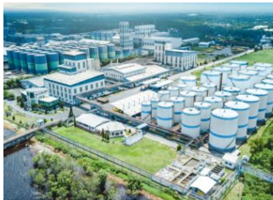
Figure 2.6 Oil Storage of PT Pacific Indopalm Industries Source: PT Pacific Indopalm Industries
