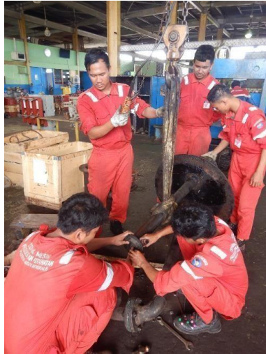
Gambar Lampiran 1: Maintenance Vertikal Sump pump
