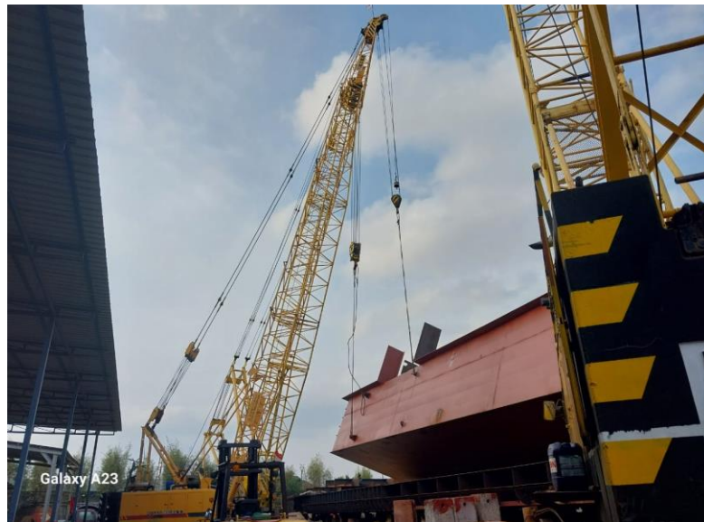
Gambar 1.3 Proses lifting ( Sumber: PT.Usda Seroja Jaya)
