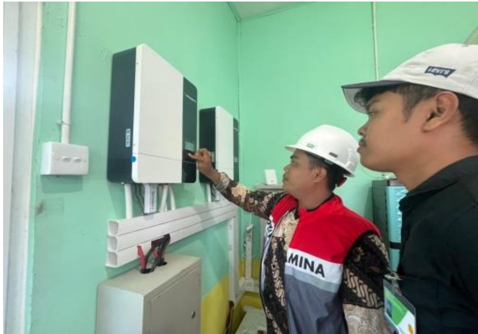
Figure 3.16 Monitoring the Installation of Solar Panels
