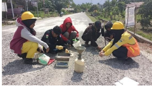
Gambar 3.28 Pengujian Sand Cone Base A
