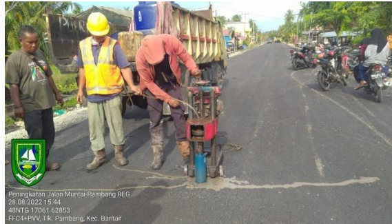
Gambar 3.37 Core Drill AC-WC
