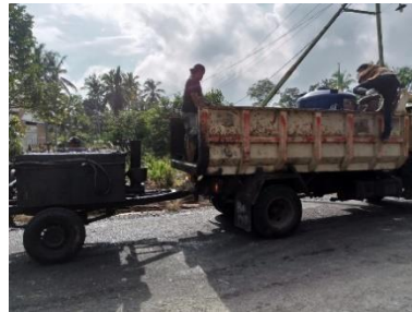
Gambar 3.15 Prime Coat
