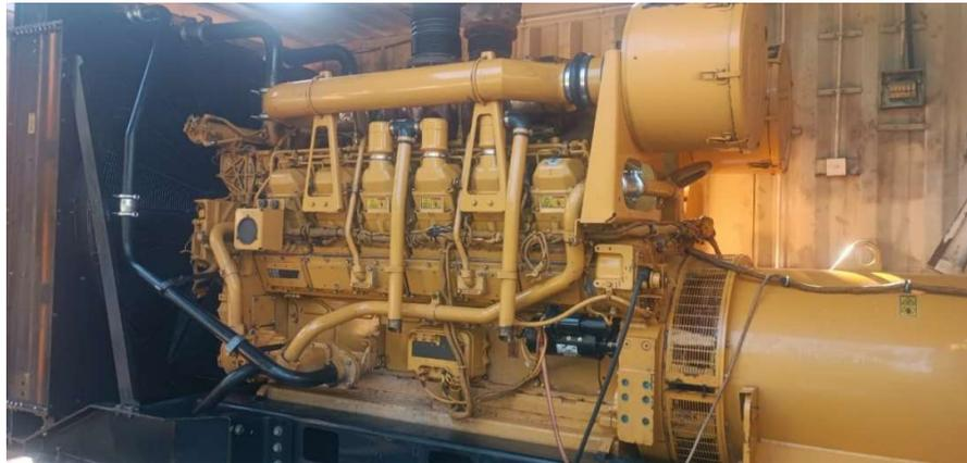
Gambar 4.1 Mesin Caterpillar Type 3512B
