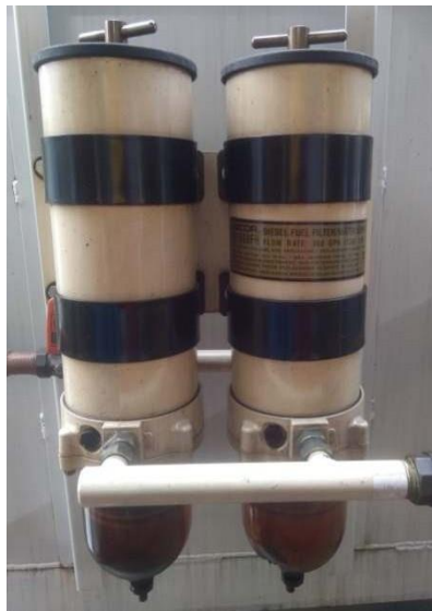
Gambar 4.4.2 Primary Fuel Filter/Water Separator
