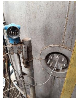
Gambar 2. 14 Pres transmitter
