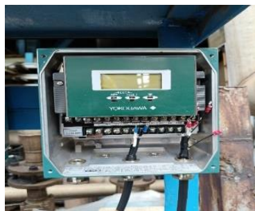
Gambar 2. 5 Connect flow transmitter 503
