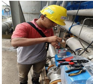
Gambar 2. 19 On off control valve
