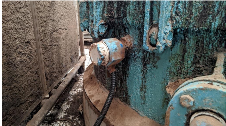
Gambar 2. 13 Pergantian kabel sensor level switch di plan refinery 1 (Sumber: Dokumentasi, 2024)
