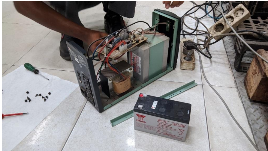
Gambar 2. 26 Pergantian baterai UPS ( Unit Power Suplay ) (Sumber: Dokumentasi, 2024)
