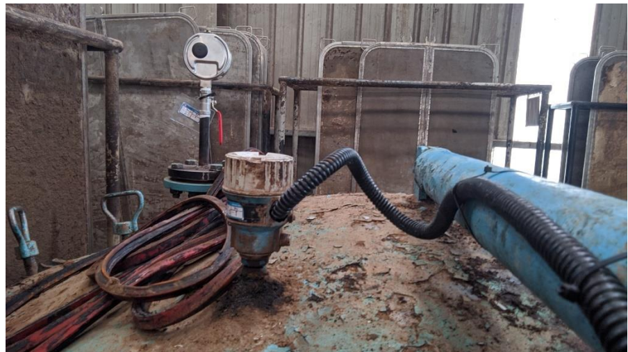
Gambar 2. 14 Pergantian kabel sensor pressure gauge di plan refinery 1 (Sumber: Dokumentasi, 2024)
