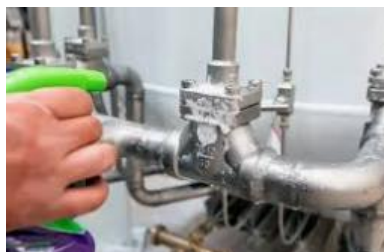
Gambar 4. 9 Leak Testing
